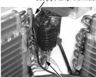
Liquid pipe temp. thermistor (TH22)
